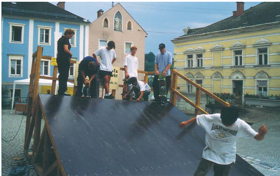
Ottensheim skater ramp construction
