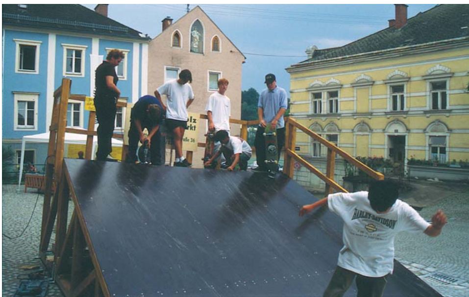
Ottensheim skater ramp construction
